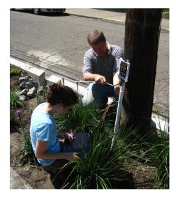
Krissy Hopkins and Dan Bain install soil moisture sensors to monitor a bioswale in Greenfield, PA. July 2012
